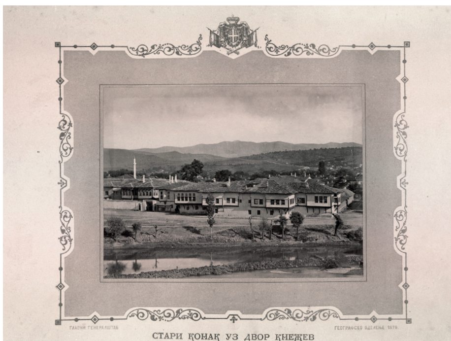
Fig. 4.1: Hafız Pasha's konak together with Bekir Bey's 1860s extension visible on the left side. Courtesy of National Museum Niš, Photo Collection, Album of King Milan Obrenović, Inventory number 13.
