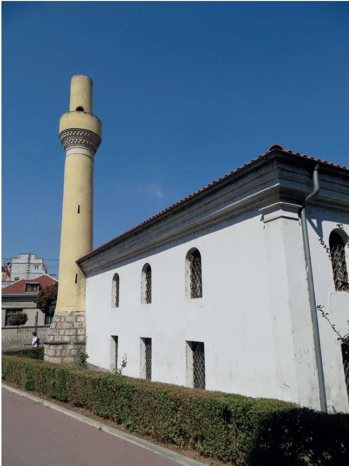
Fig. 7.1: Islam Aga Mosque with minaret missing its cone shaped roof. Meanwhile it has been restored. Photograph by Florian Riedler, 2012.
